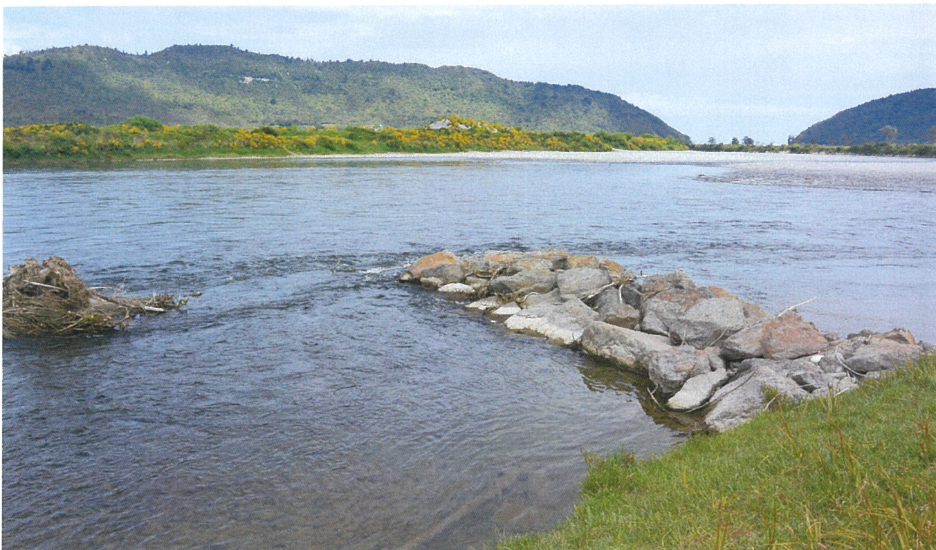
Coal Creek spur, looking downstream. 30 Oct 2017.
